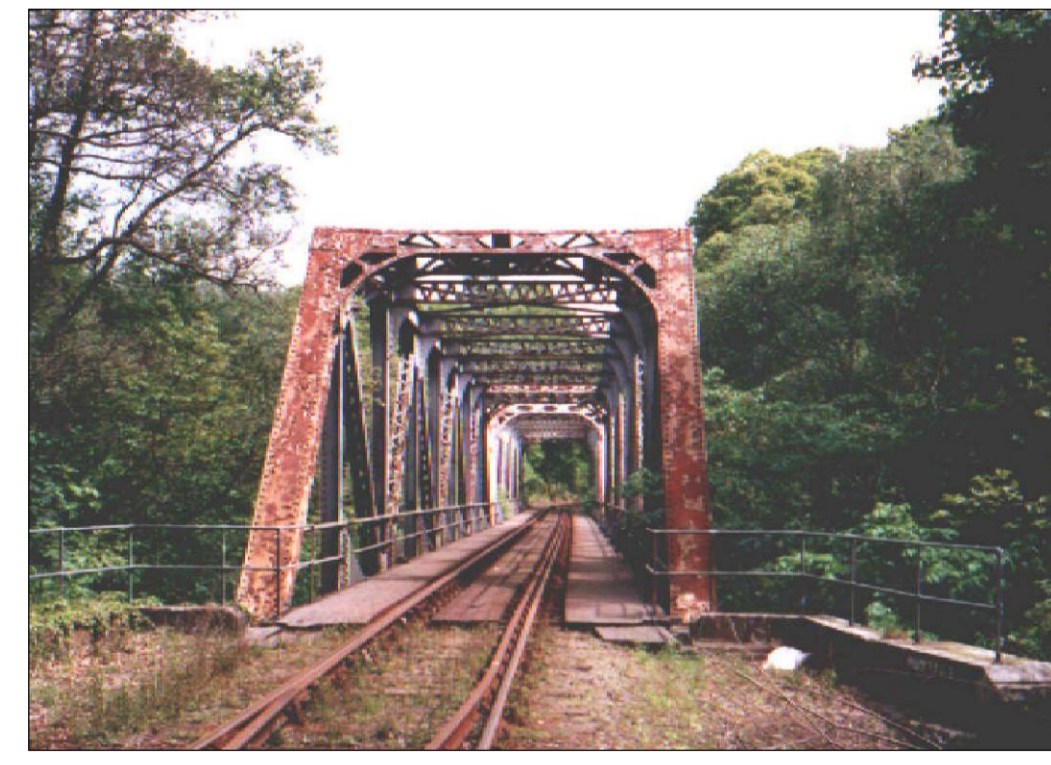
PHOTOGRAPH AT TRACK LEVEL UNDER BRIDGE MBW2.82
